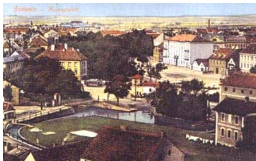
Fig. 7: The Millrace in Senovážné Square. The view from the beginning of the 20th century.
