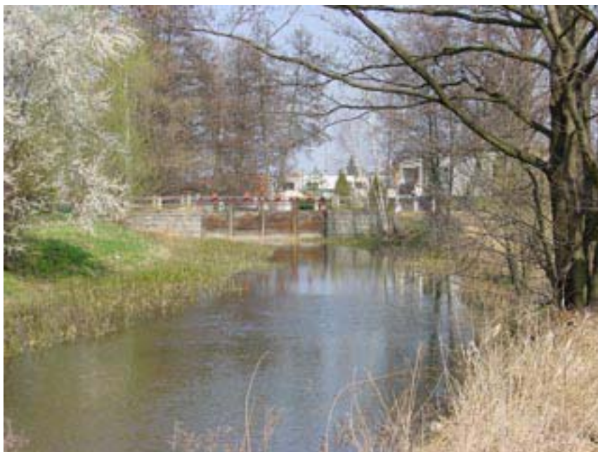
Fig. 5: The Dam on the Millrace which regulates the amount of flowing water.
