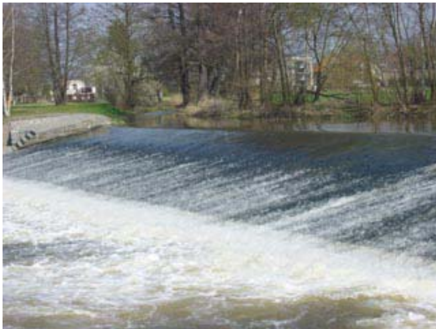
Fig. 2: The Great Weir at the Red Yard in Mladé. The Millrace separates the Malše branch just above the weir..
