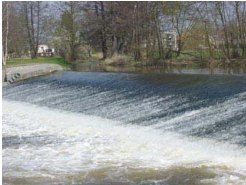
Fig. 4: The Great Weir at the Red Yard in Mladé. The Millrace separates the Malše branch just above the weir.
